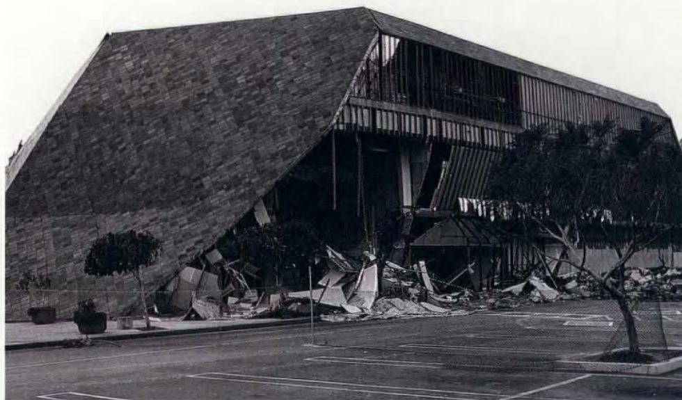
Department store wrecked by column/slab joints wrenched apart
