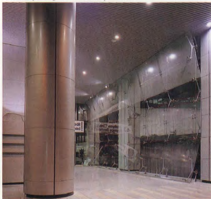
T.R. Hamzah & Yeang have recently completed this structural glass curtain wall at the headquarters of the South East Asia Development Corporation in Kuala Lumpur. Engineers were Whitby and Bird
