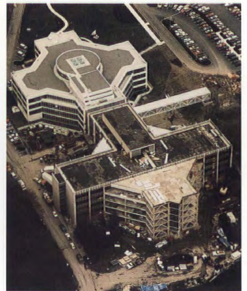
GTE exteriors (top and above) show completed building concealing incorporation of original 1960s structure. Progress shot (right) shows original structure gutted in foreground
