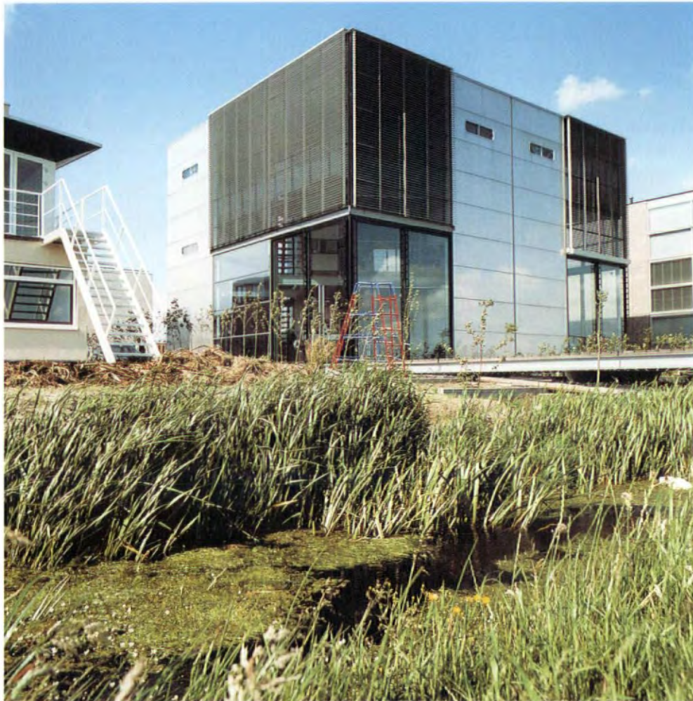
The Pesman house, Delft, features a diagonal servicing wall within a rectangular plan (this page) with alternate glazed and pressed metal cladding panels. 1987 Nieuwegein Technology Centre (opposite page) uses same technique on larger scale
