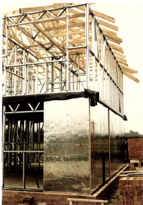
(Below) Steel framed house during construction showing celotex insulation
