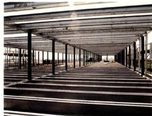
Terrapin Matrex cold-rolled beams during construction
