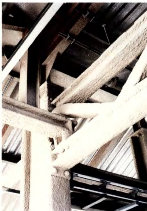
Terrapin Matrex cold-rolled beams during construction
