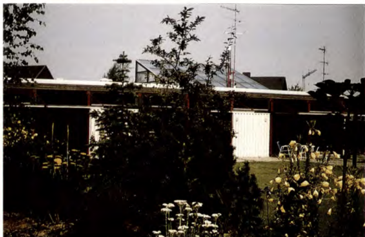
Schulitz House, Braunschweig, 1985. Standardised lightweight components on a timber frame with ingenious "up and over" insulated panels - open for the summer (below) and closed over the windows in winter (bottom)
