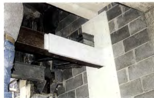
Fire protective coatings by Mandoval – steel construction spray coated (below left) and clad with pre-fabricated panelling (below)
