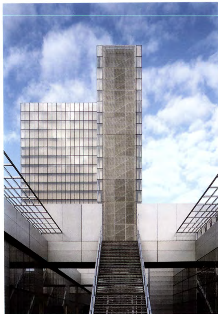
Above The four "open books" of Perrault's new library. Left and opposite page bottom The building's towers have been enveloped in "the most transparent glass possible" – Securiflam laminated glass. Opposite page top Transverse section and longitudinal section, below
