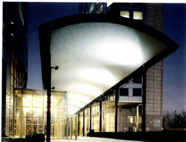
ING and Stibbe Twin Towers in Amsterdam
