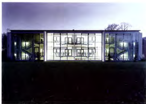
Gymnasium, Usingen by Bremmer Lorenz Frielinghaus & Partners
