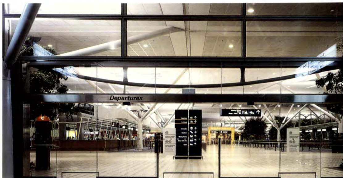
Above View of the full height glazed walls and white color-bond roof, with six metre eaves – to protect the window walls from the harsh Queensland climate.
