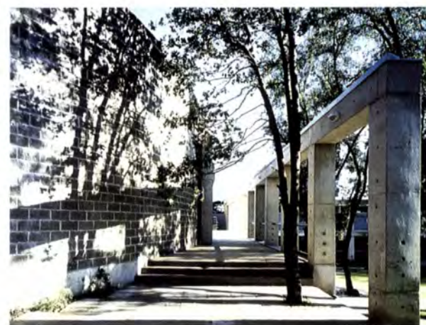
Opposite page Interior of building showing strong minimalist sympathies and flexible spaces. Above top Entrance between carefully preserved trees and the strong curved wall of the outside of the auditorium. Bottom The concrete colonnade continues the strong geometrical grid of the facade of the building to the right of the entrance. Again the architects have kept existing trees to soften the formal built environment and to create dappled light
