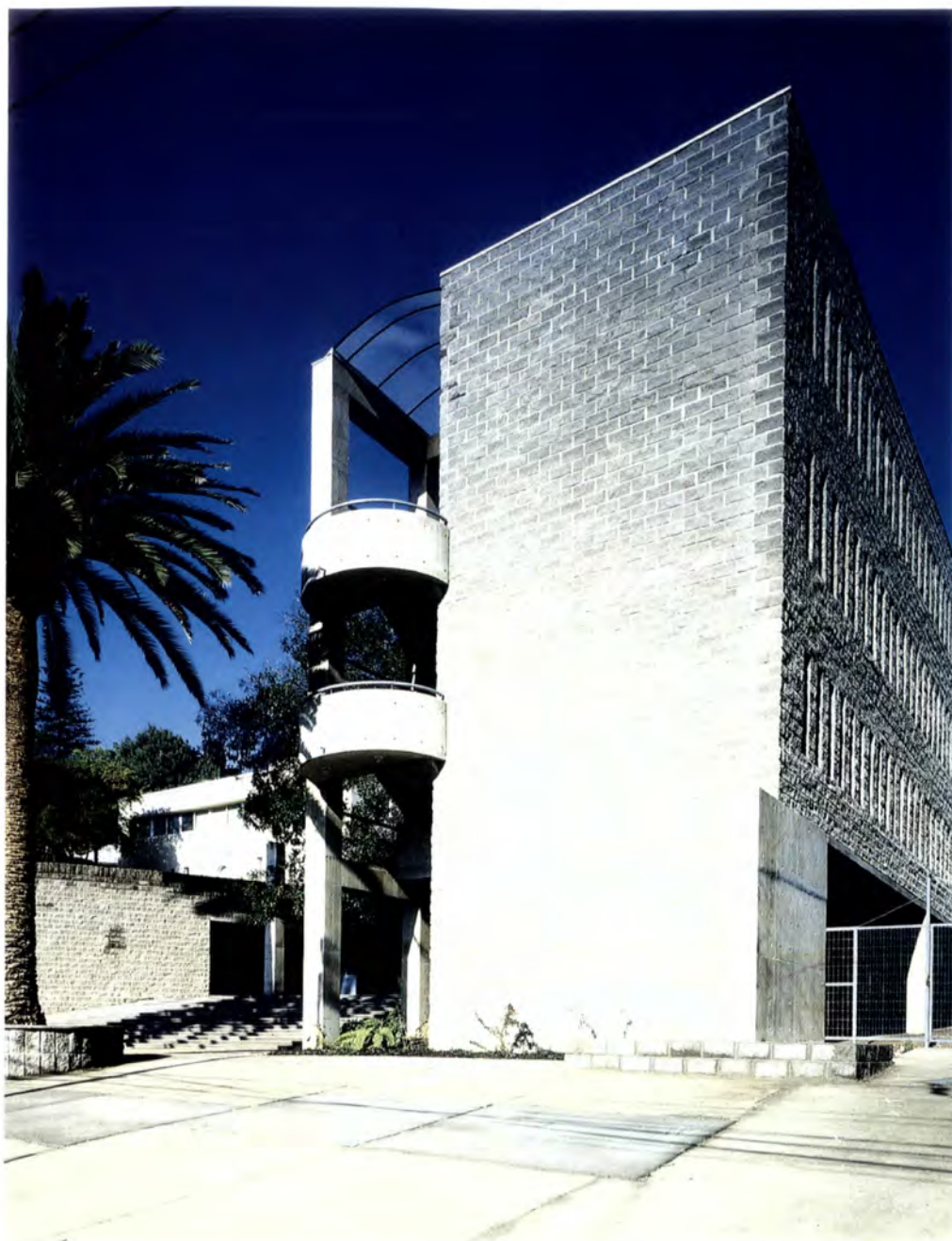
Left The street end of the four-storey classroom block. Circulation space can be outside the main body of the building due to the pleasant climate of this seaside resort town of Viña del Mar. Below top The "main activities courtyard" designated as a space for student meetings. Below bottom The triangular volume between the existing house and the classroom block contains the cafe, showing how the interior space echoes the geometry of the project as a whole
