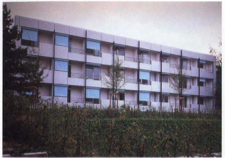
Above left and right The exterior was improved by the addition of steel structures to the windows, colourful sunshading and a programme of planting
