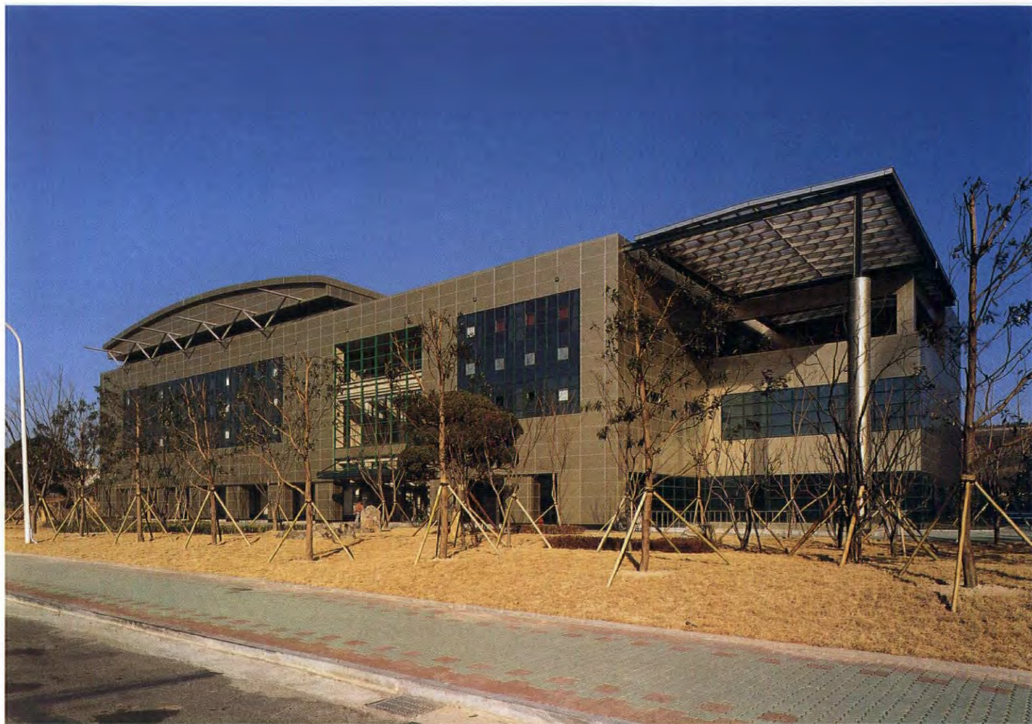
Above The Centre acts as an oasis in a harsh industrial environment. The building is clad in corrosion-resistant bronze-coloured aluminium. Right Ground floor plan
