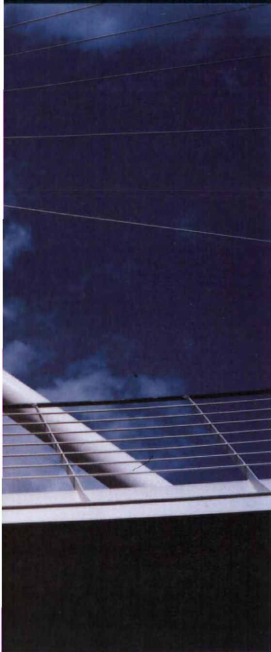
Left View of 41-metre, cigar-shaped pylon. Below Axonometric. Bottom Lighting plays an important role in the overall design concept. Bulkhead lamps are built into the cable anchorage housing along the centre of the main deck
