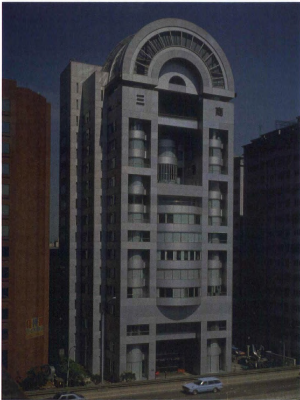
Left The barrel vaulted roof appears to float above the aluminium clad facade. Bottom left The full height atrium is overlooked by terraces on every floor
