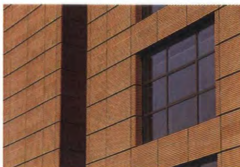
Over the years the RPBW have refined their use of terracotta cladding. At Lodi terracotta has been used to refer to the agricultural context of the site. Middle Detail of the upper edge of the Lodi facade. Bottom Elevation and section of typical bay
