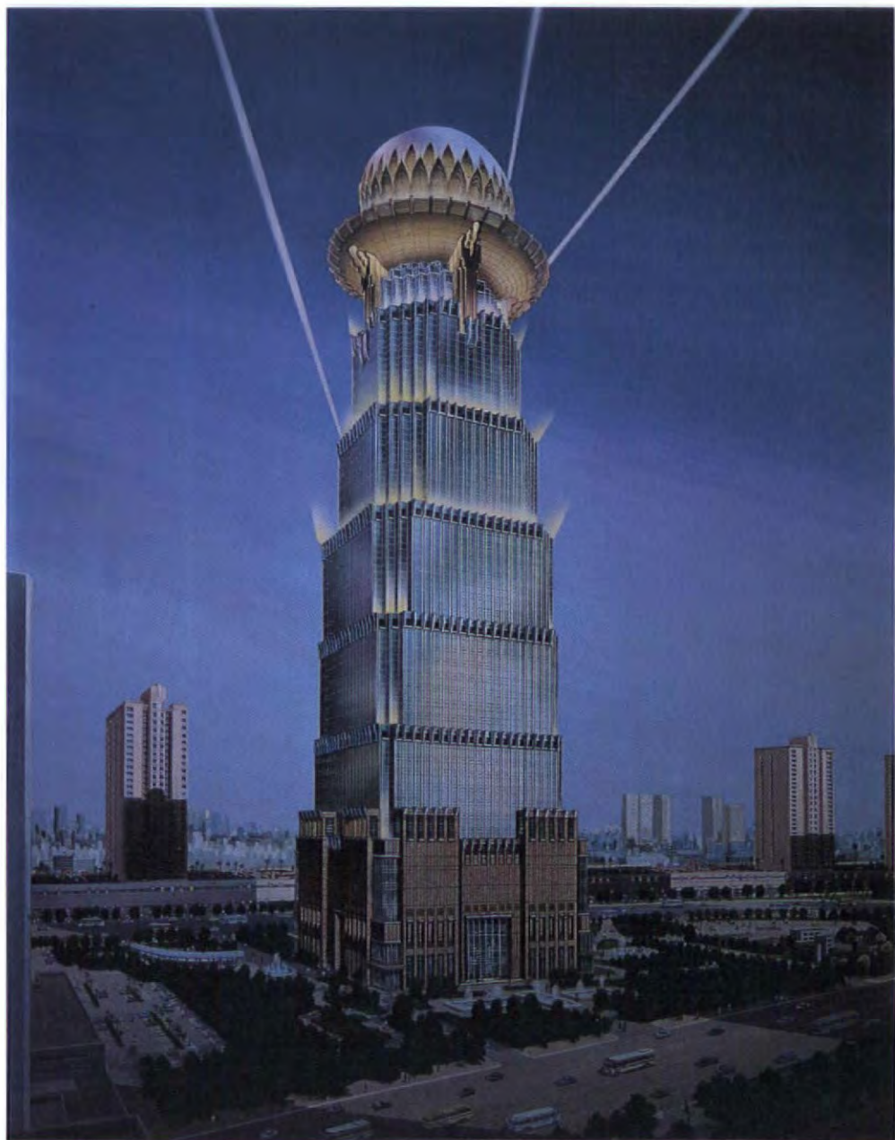
Left A glass office tower supports a dish containing a geodesic dome in the form of a Lotus flower, within which is a restaurant. The whole building sits on a granite clad retail podium. Bottom Longitudinal section
