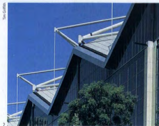
2: Profile of the convention centre's external space-frame roof
