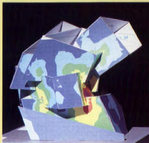
2: The proposed extension to the Victoria & Albert Museum in London designed by Daniel Libeskind represents a new dynamism in structural engineering. Coloration of model shows computed stress levels in the structure
