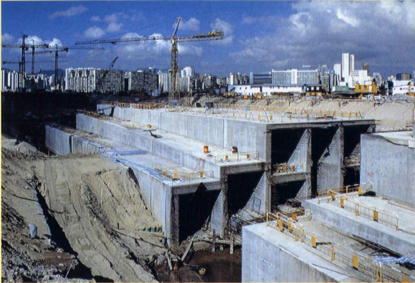
4: Kowloon Station cut and cover tunnels under construction. Four railway tunnels plus ventilation tunnels and sidings
