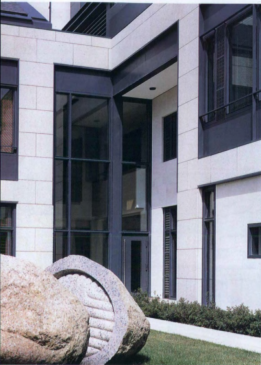
1: Courtyard elevation looking into the inner hall
