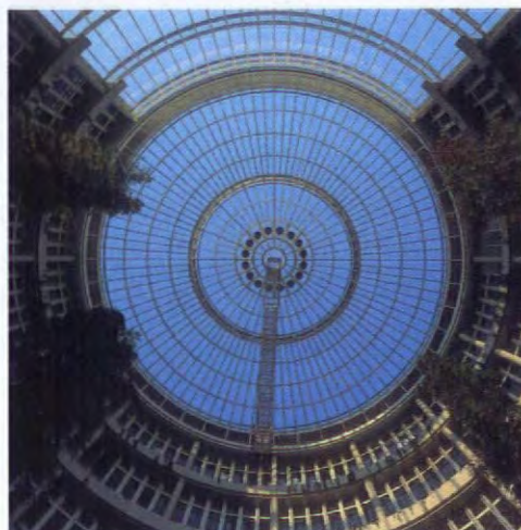
Internal maintenance gantry Schering AG, Berlin
