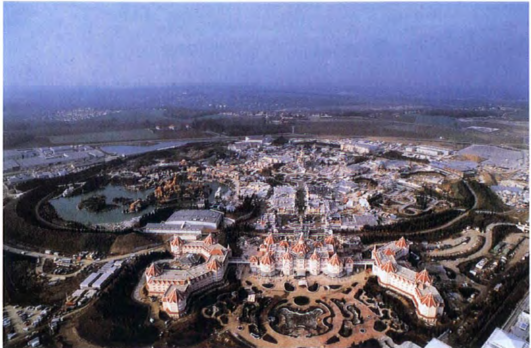
1: Aerial view of Disneyland, Paris under construction
