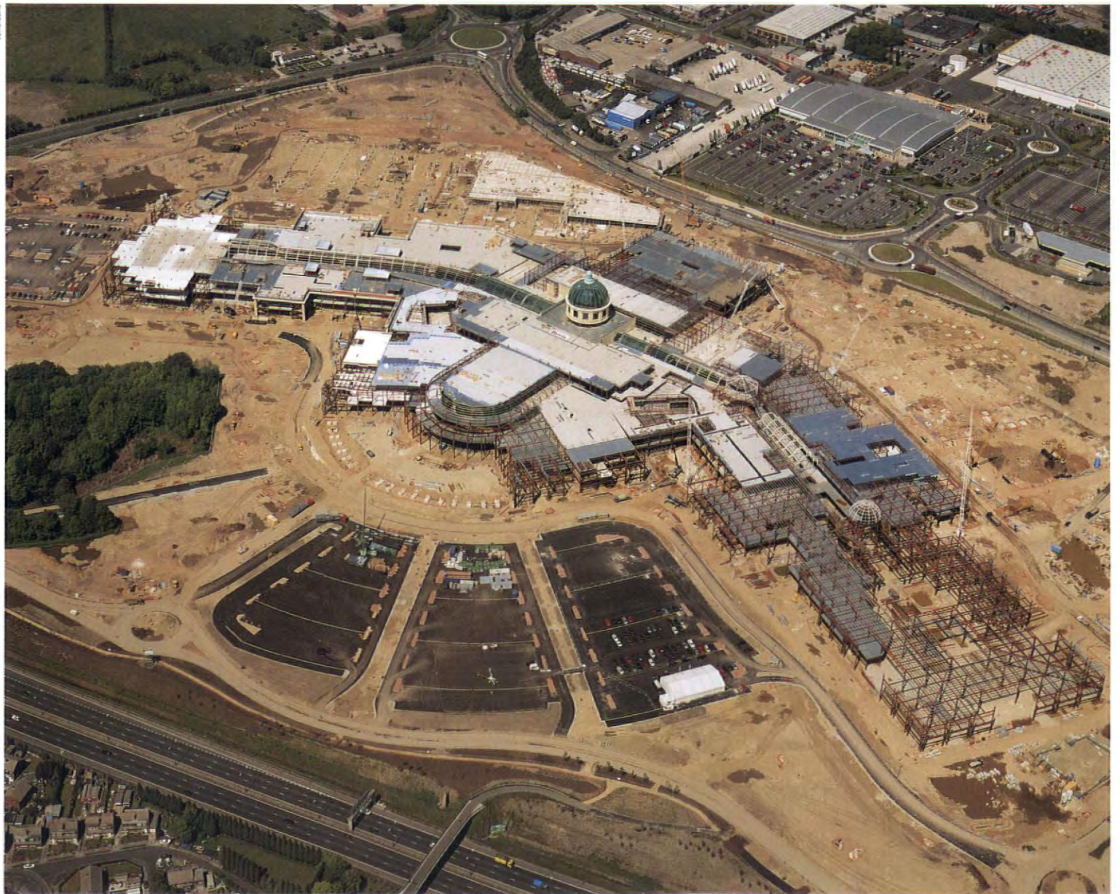
1: Aerial view of the Centre during construction
