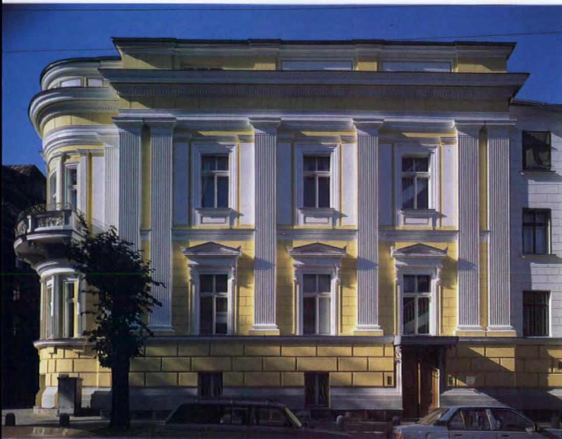
1: Elevation of the embassy alongside A Pumpura iela
