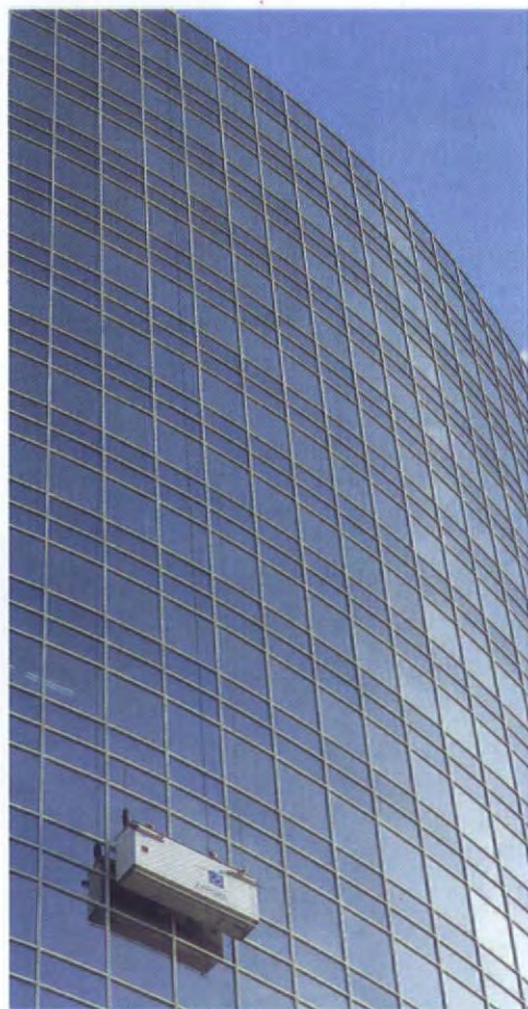
Building maintenance unit Ventura office block, Eschborn/Frankfurt
