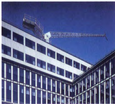
Building maintenance unit Trigon, Berlin
