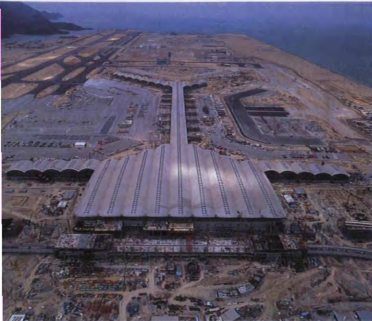
The 39-gate terminal at Foster's Chek Lap Kok airport has a 490,000 sqm concourse and gate area which narrows and stretches 1.3 kms before it splits like a swallow's tail
