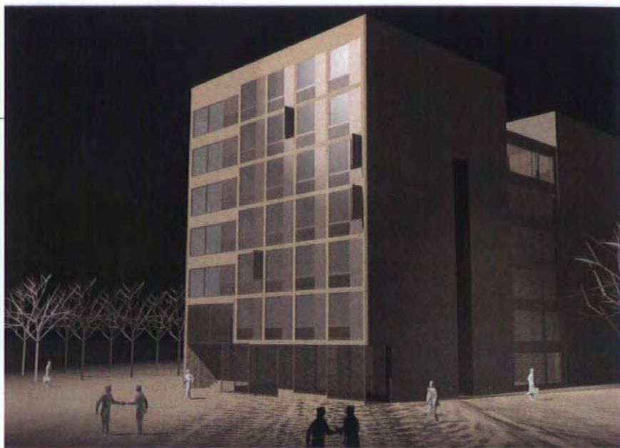
Computer image showing the reinforced concrete sheer walls and single and double glass infill walls
