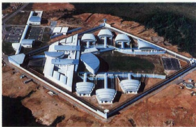
Far right and facing page: The use of pre-cast concrete cells is a fairly recent innovation, but can cut the critical mass required in a facility to a lower number of cells
