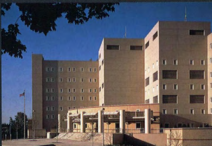
Left: NBB's Federal Detention Centre, King County, Washington, USA – a 677-bed facility which cost US$56,000,000
