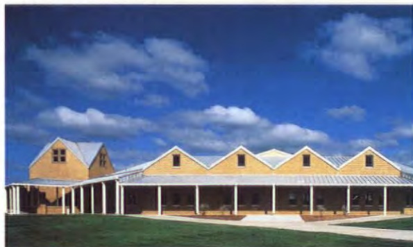
Federal Bureau of Prisons, Three Rivers, Texas, USA
