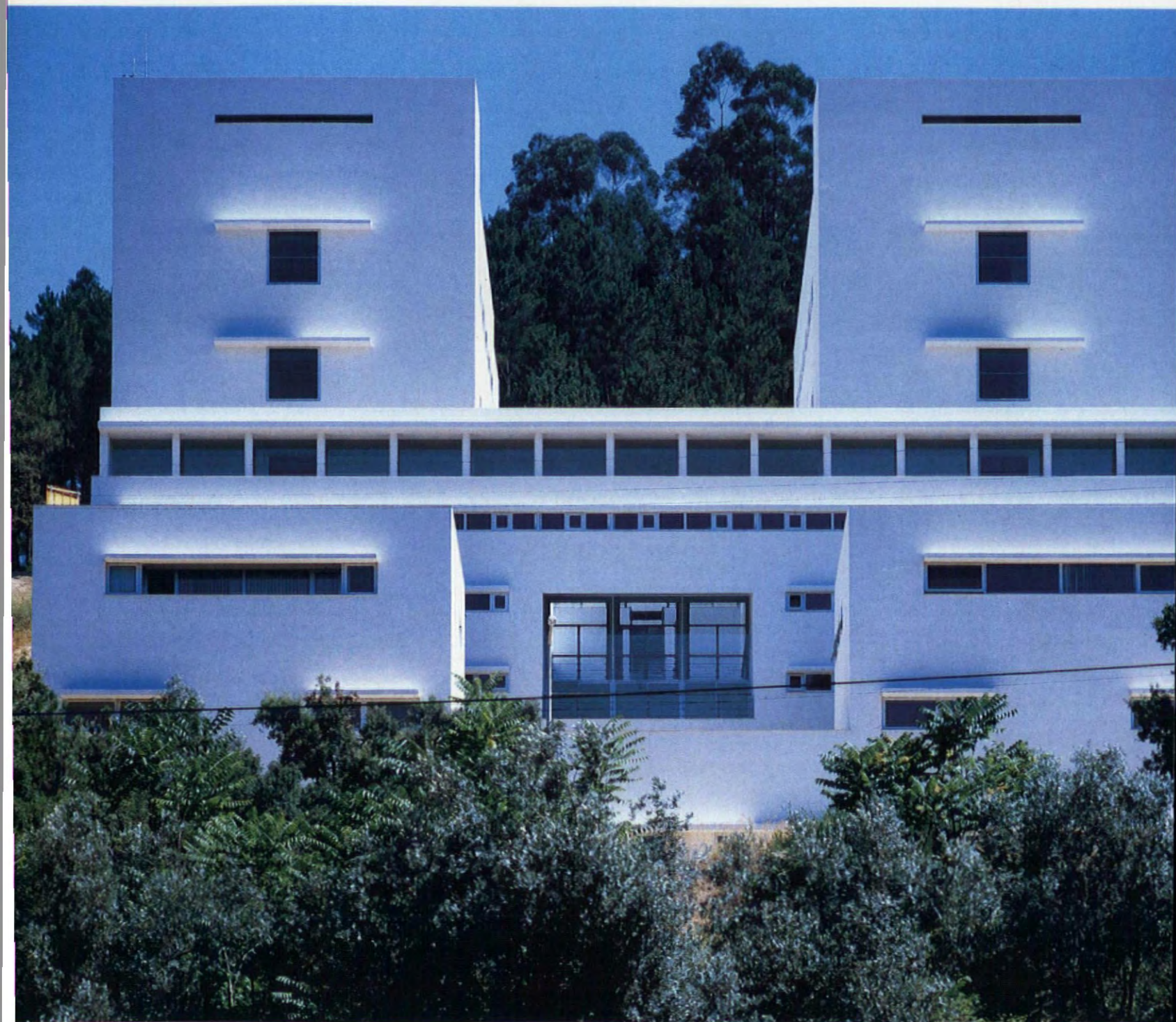
Partial view of the western end of the School of Electrical Engineering showing the special laboratory institutes in the foreground, backed by the circulation gallery and transverse teaching volumes
