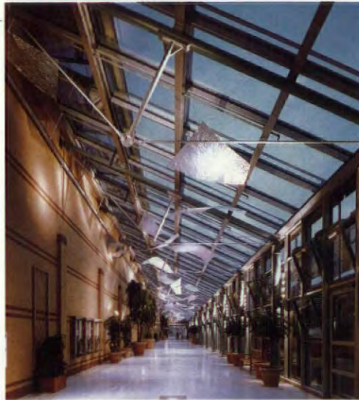
1. Magistral (large view): The glazed "magistral" constitutes the light-flooded "pedestrian thoroughfare" of the Marzahn Hospital. Low-emissivity THERMOPLUS Neutral glass is combined with the Gartner Integrated Facade featuring structural members that carry water for cooling in the summer and heating in the winter.
