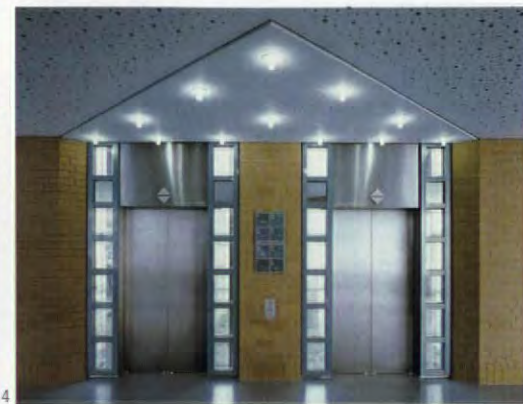
4. Elevator Shafts: The walls of elevator shafts and fire doors to stairwells and between wards feature PYROSTOP glazing in compliance with fire-resistive ratings F 90 and F 30.
