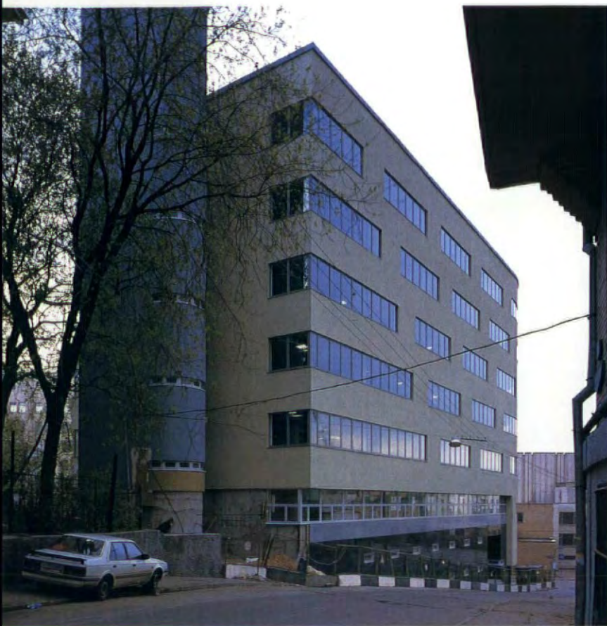
The fire-escape staircase at the rear is linked to the building at each level by covered bridges
