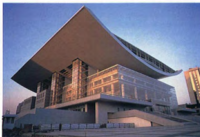
Jean Marie Charpentier et Associés' Shanghai Opera House is a flagship for aluminium roofing in the South-East Asia. The region's construction industry is one of the world's major users of the metal
