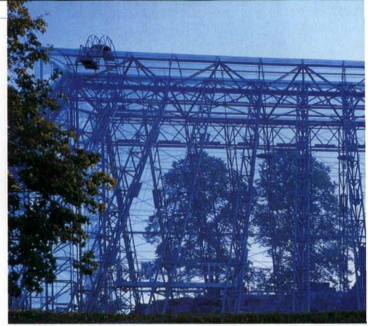
The Hamar Cathederal protective structure – the curved vaulted roof is open in the centre to ventilate the interior.
