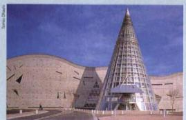
Above and left: Kisho Kurokawa's glass cone at the Amber Hall, Kuji City, comprises untreated strengthened float glass – sunshading is achieved with white punched aluminium screens and fancoil units
