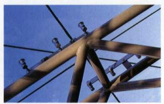
Left: Detail showing the extremely complex bolt connections and structure as seven panes meet in the same place
