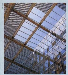
The Herne-Sodingen Academy by Jourda and Perraudin, Duisberg, Germany. HL Technik AG's glazed hall is hung from a wooden support frame and incorporates photovoltaic cells which are positioned to allow maximum light through the roof.
