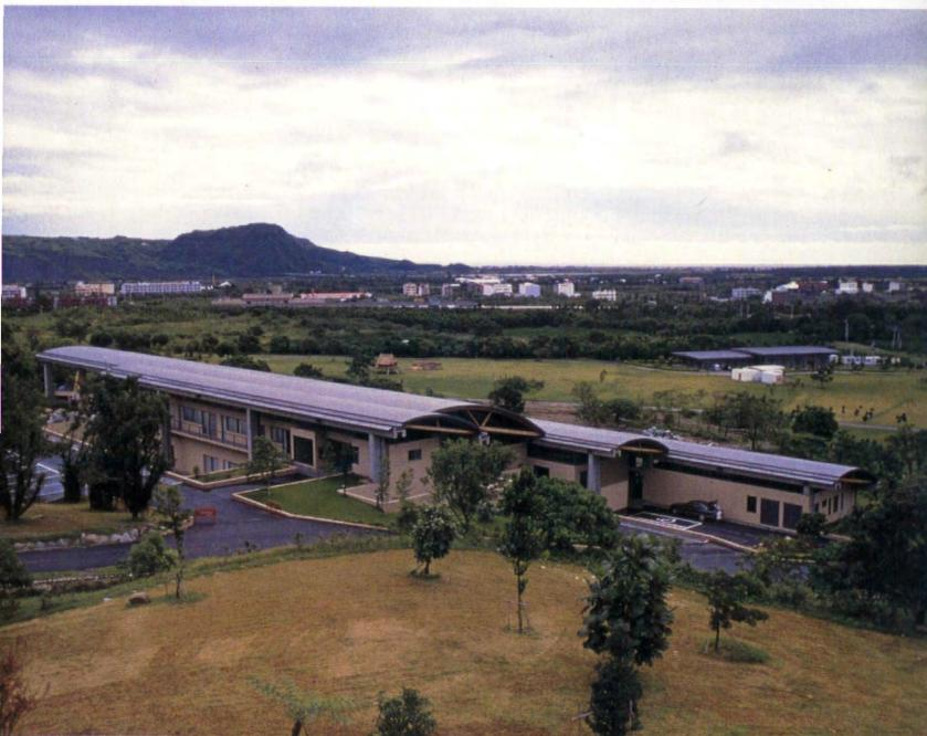
for climatic reasons, and to create a warm space. The bowed upper and lower sections are designed to resist typhoons, to which the region is prone.
