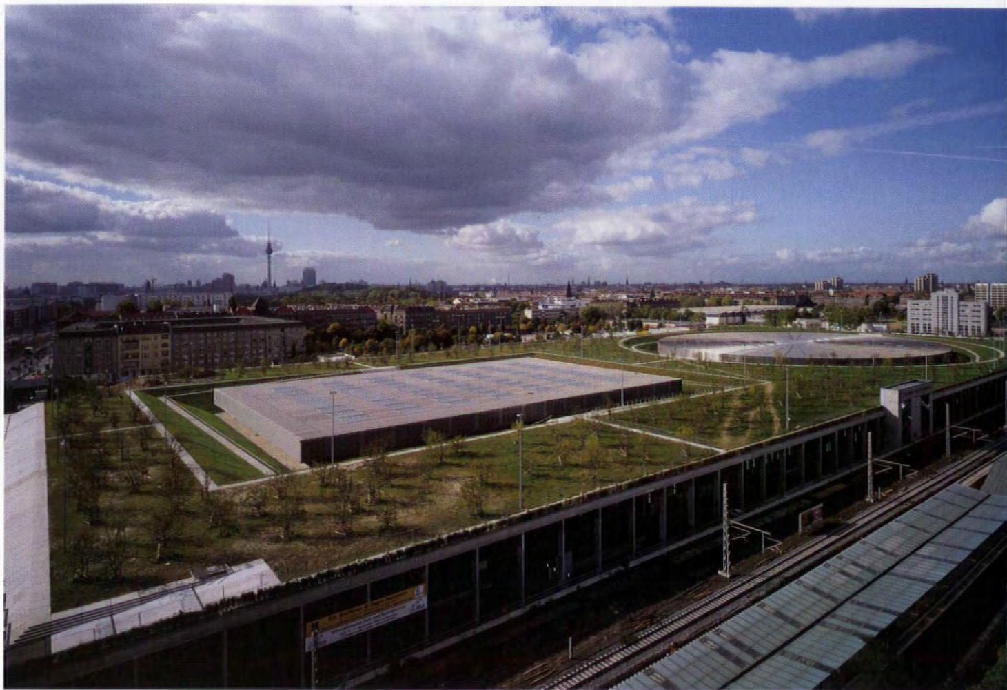
Above: The rectangular pool and circular velodrome are sunk into the landscape, and clad in glittering steel mesh
