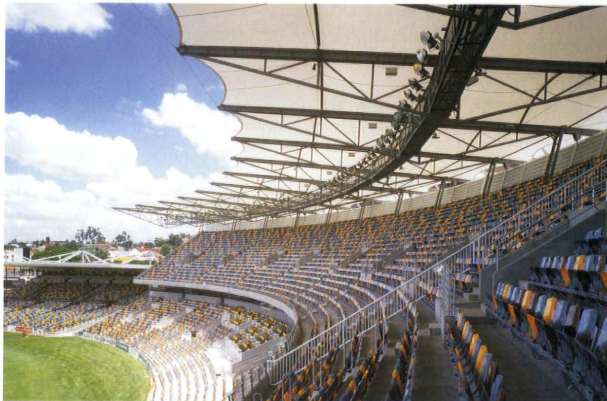
Left: Daryl Jackson's new stand at Brisbane's Gabba Cricket ground. Jackson cites "conventional technology for the fabric, innovative steel engineering for the structure; reducing cost by fire protecting the steel, and through small scale component assemblage" as key features
