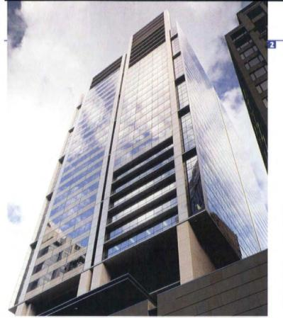
The 30m-high void beneath the tower is partially filled by a 12m-high glass box containing the lobby and public courtyard 2 363 George Street is held aloft by brace-free steel columns which act as stilts which act as stilts
