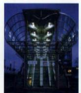
curved bullet resistant laminated glass, curved laminated solar control glass, curved non-reflective glass, curved fused glass
