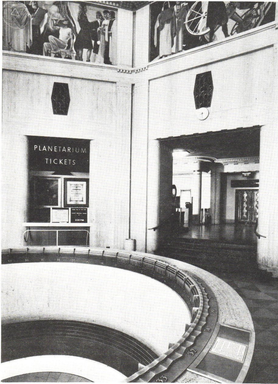
Foyer looking into pendulum pit.
