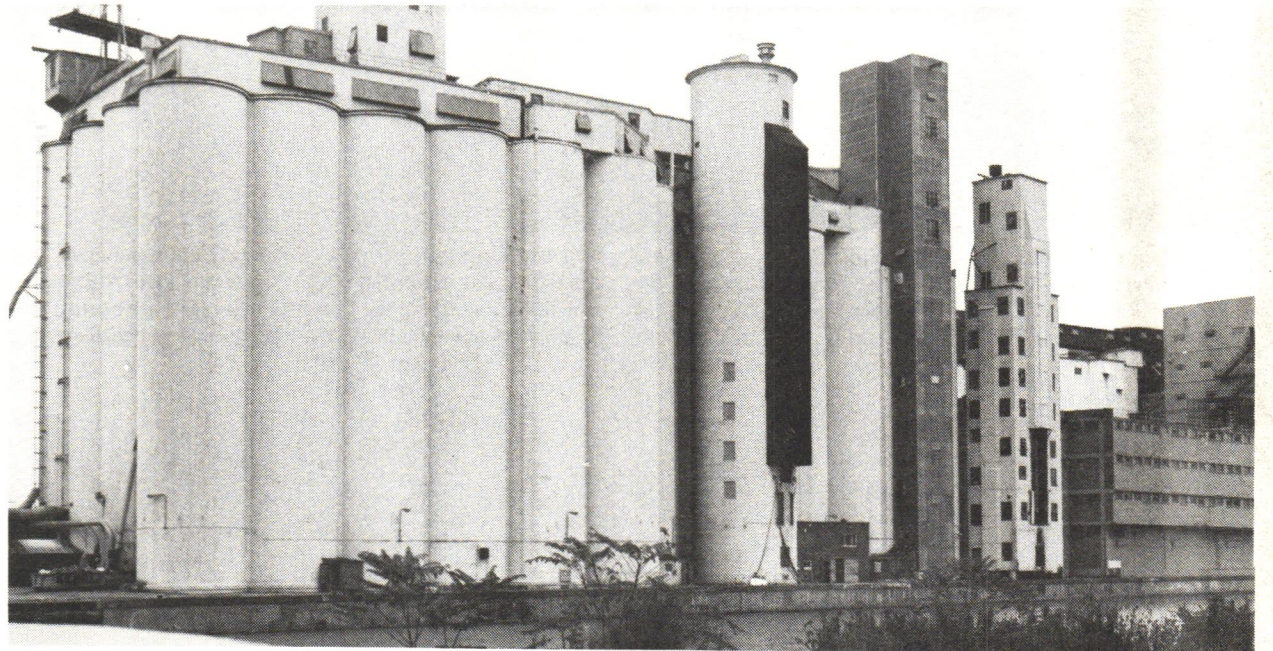
A gropian monument as it stands today: the Ex-Washburn-Crosby elevator in Buffalo, greatly extended on the left, but the dark “marine tower” (center of the three) is the same tower as shows in Gropius’s illustration
