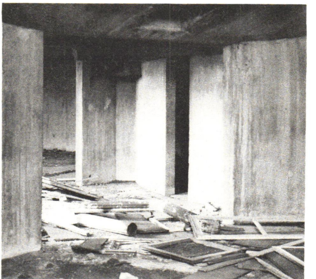
Catacombs of the Modern Movement; the circular rooms and segmental "interstitials" that housed conveyors and spouts in the bin-bottoms of the 1925 Marine-"A" elevator in Buffalo; secret spaces that Le Corbusier could have designed, but didn't.
