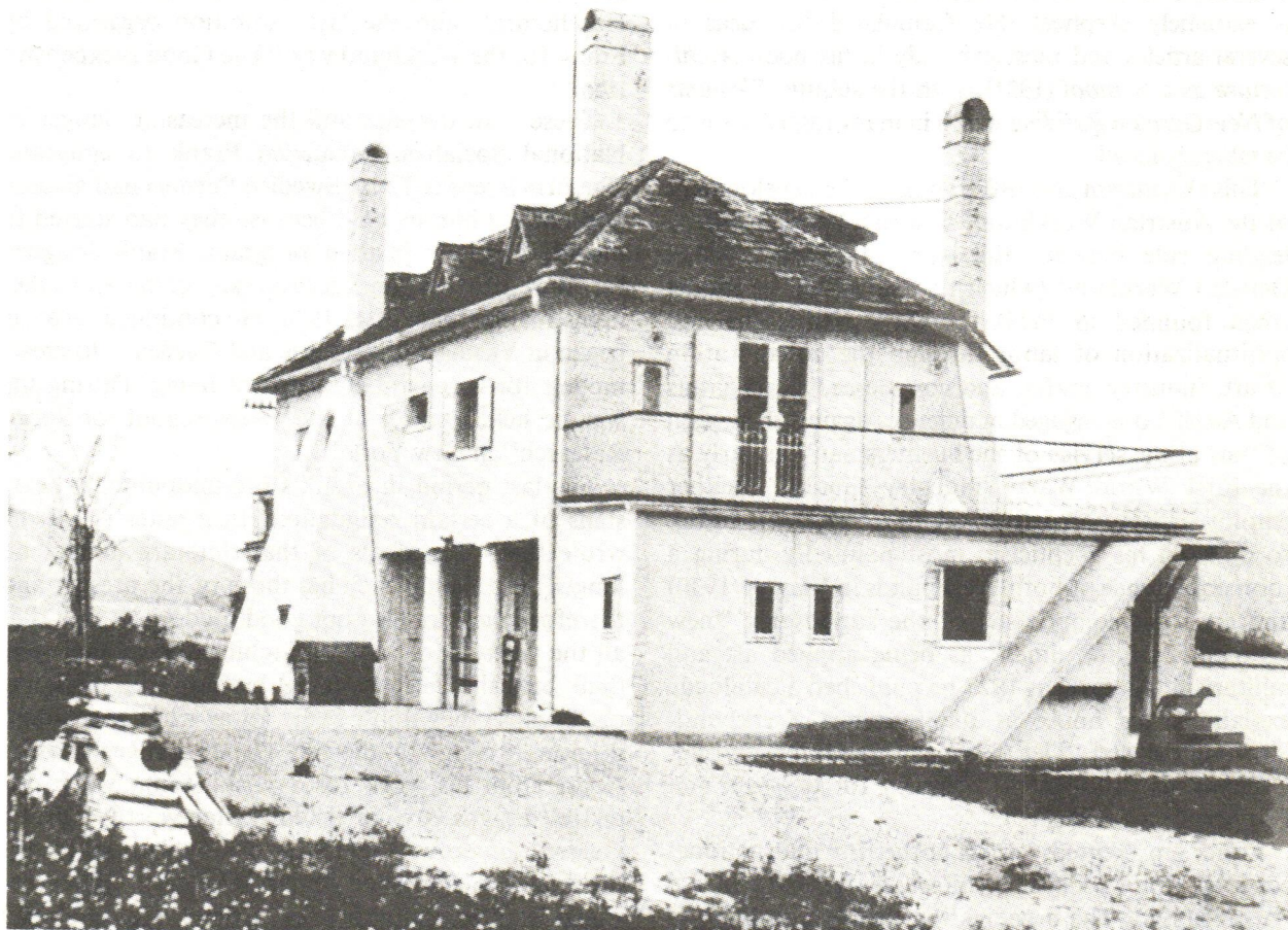
Josef Frank, Residence in Pernitz , Lower Austria, 1914.
