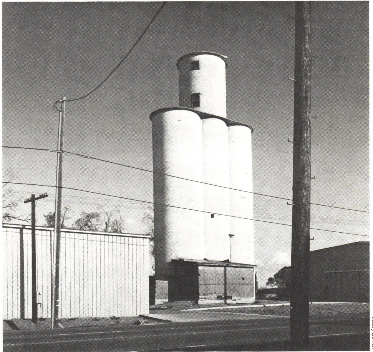
Confusing Cylinders: what appear to be simple cylindrical containers of grain can deceive the unwary observer—not only do the windows indicate the presence of machinery, not grain, in the
