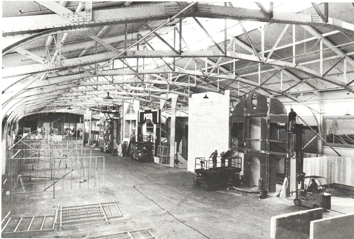
The Strada Novissima under construction. One of the indispensable scissor lifts is on the right.
