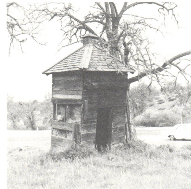
A four-way hip roof with cupola is the distinguishing feature of this stage coach inn rest stop near Jolon, California.
