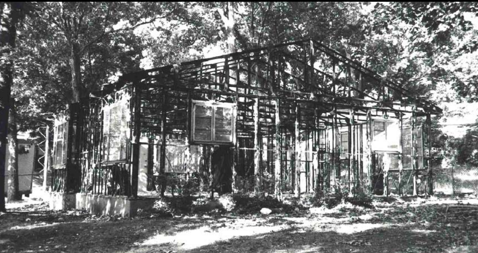
Only the metal shell remains, looking southwest. —Cynthia Liccese-Torres, June 6, 2006
