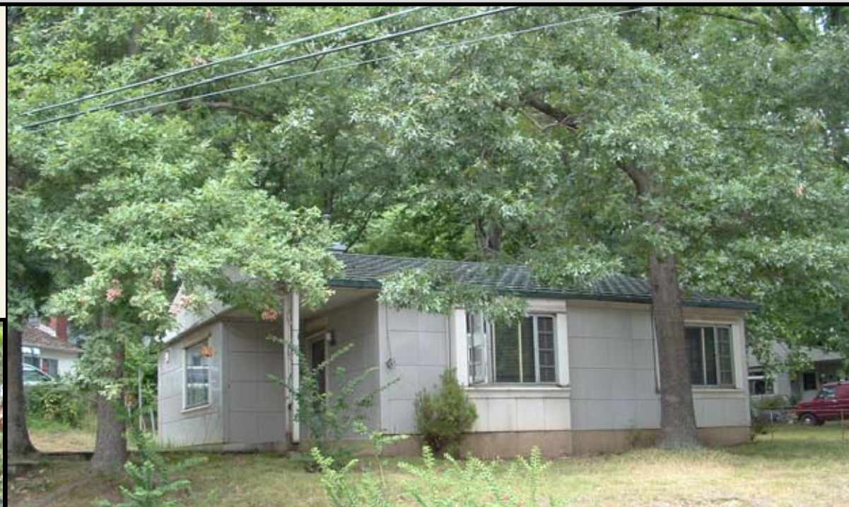
Front elevation of the Clifford M. Krowne Lustron House on its original lot, 5201 12th Street South, Arlington, Virginia. A neighboring Lustron still stands at 1124 South Frederick Street (at far right of photograph). —Cynthia Liccese-Torres, August 2005
