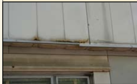
Detail of rusting at base of vertical panels along the gable ends. —Todd Zeiger, May 3, 2006
