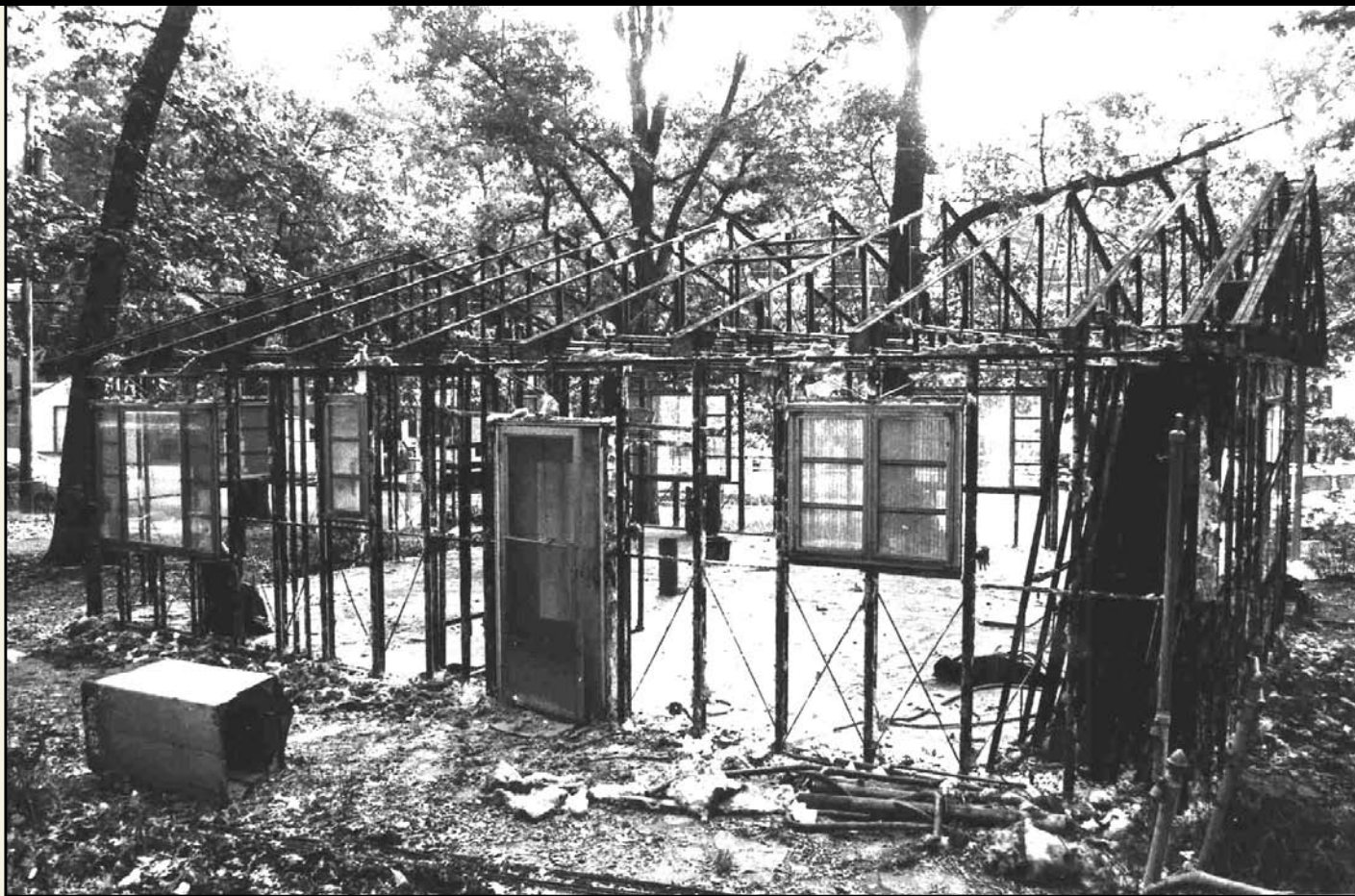
View of rear (west) elevation, looking east. —Cynthia Liccese-Torres, June 6, 2006
