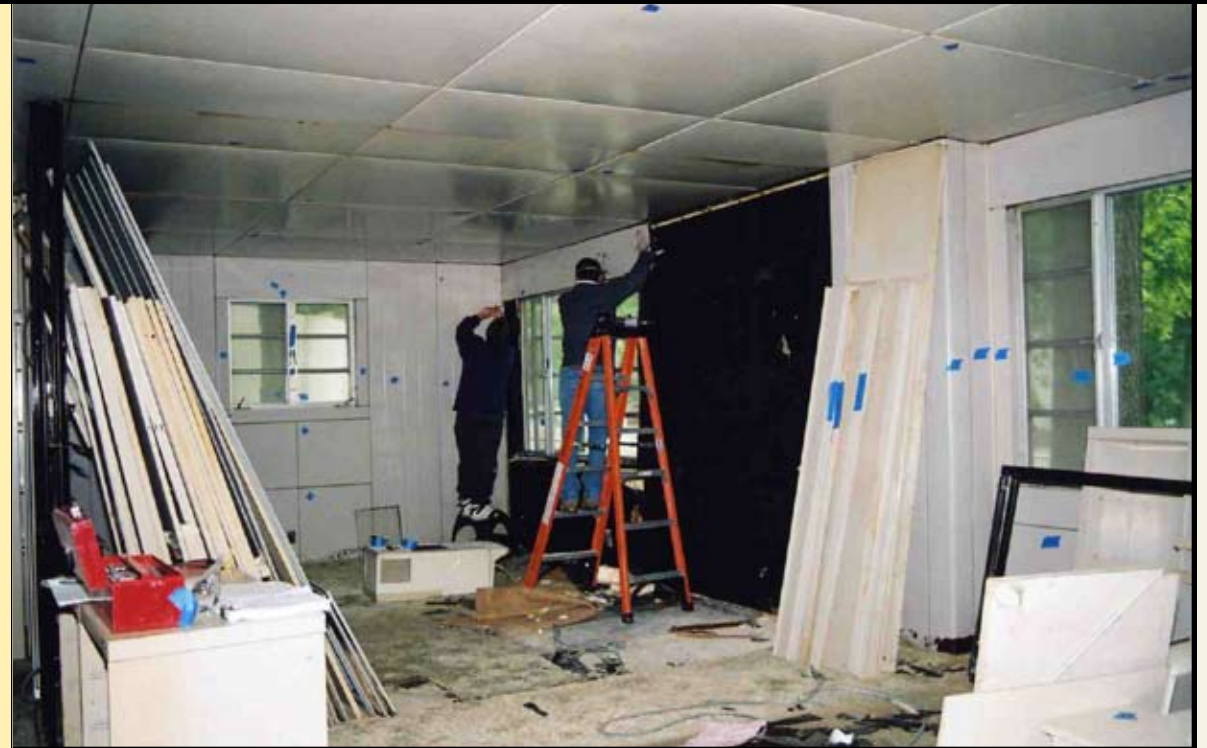
Interior wall panels being removed along the front wall of the master bedroom. —Victor E. Muniec, May 5, 2006
