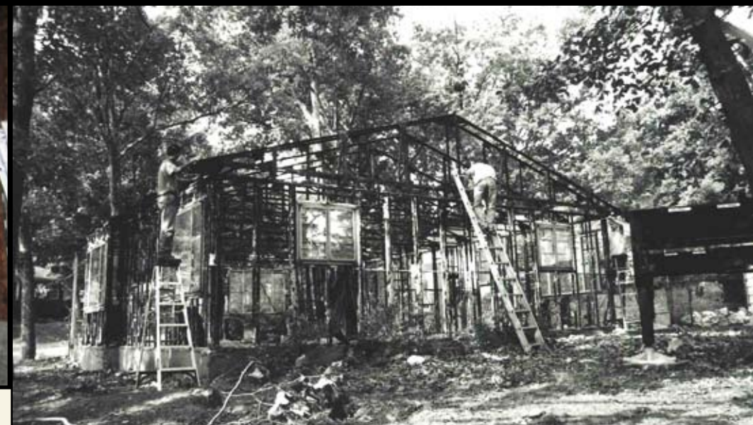
Securing the first roof truss to be lifted by the crane along the northern edge of the house. This process was made easier by three crew members – one on each end to loosen the corner bolts and one in the middle to secure the truss to the crane anchor. —Cynthia Liccese-Torres, June 8, 2006
