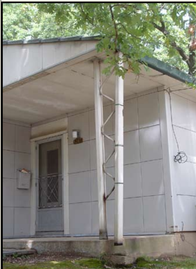
Detail of original front porch pier and gutter. —Cynthia Liccese-Torres, August 2005
