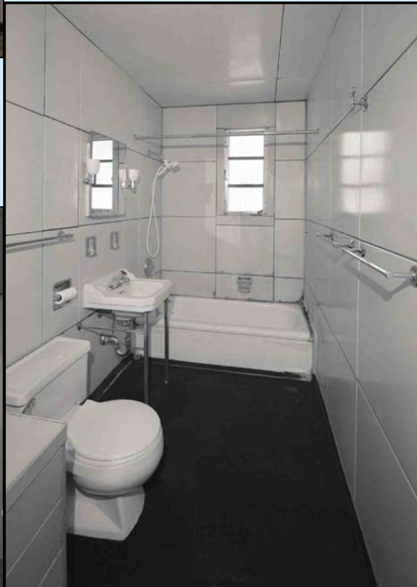
Bathroom of the Krowne Lustron House. All features are original, with the exception of the toilet, faucet, and shower head. —Photographed by James W. Rosenthal, Historic American Buildings Survey (HABS), National Park Service, March 2, 2006
