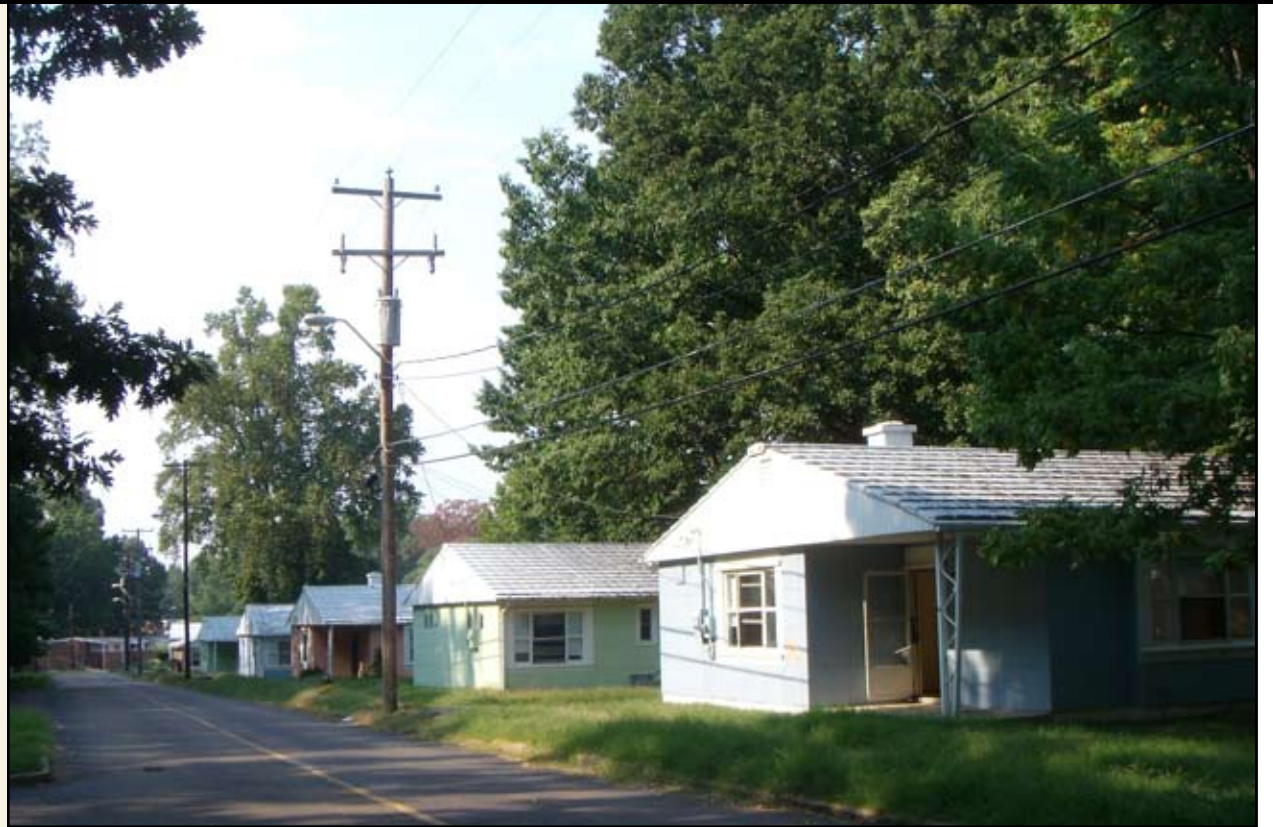
Enclave of original Lustrons at the Marine Corps Base in Quantico, Virginia. This subdivision of Argonne Hills in the central portion of the base was removed in October 2007. —Cynthia Liccese-Torres, September 26, 2007
